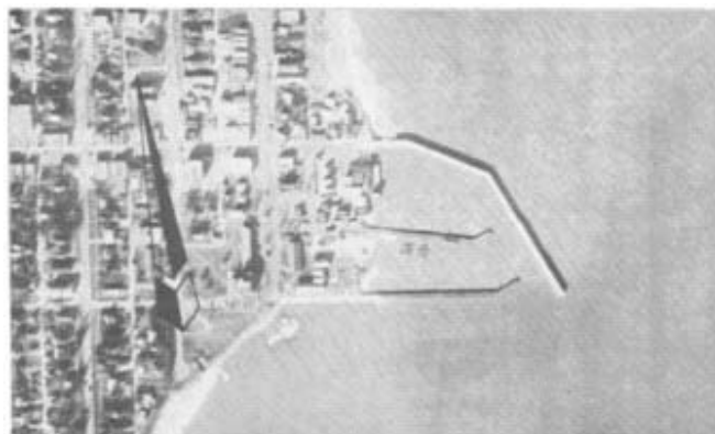
Gimli. The pole lamps have electrical outlets attached. The north sea wall has been increased five feet.
