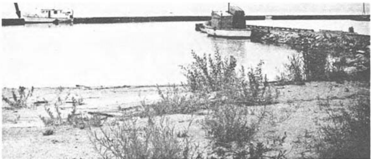
Hnaua. The fact that the hull sticks above the wharf illustrates the poor protective qualities of this harbour. The new inside wharf is the best location but its size is limited.
